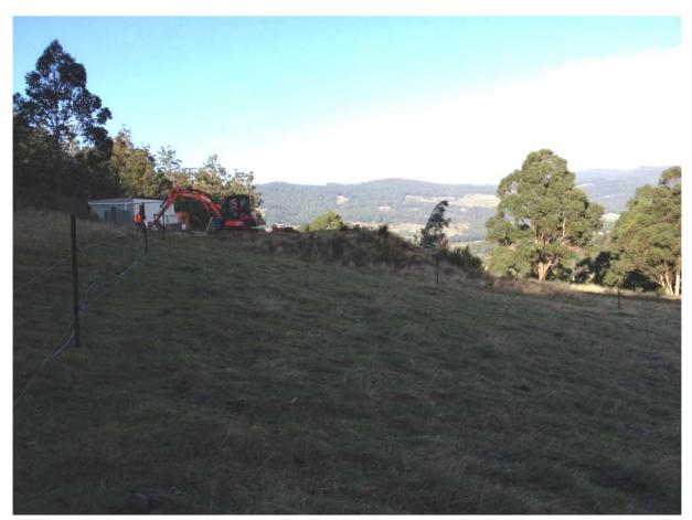
Plate 5 (above). View south and cross-slope towards the pad for the house, showing the (presumably uncontrolled) fill from the excavation placed by a previous owner. The slopes in the foreground are flattening from  $12 - 10^{\circ}$ .
