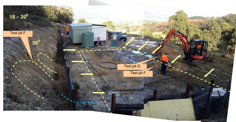
Plate 9 (above). View south southwest showing the proposed house site (yellow dashed line; approx. only), previously-dug auger holes for piers (arrowed), test pits F and G, the steel-posted and undrained timber retaining wall (blue dashed line shows water flow), the 350 batter slope behind, and two very small rotational landslides on the batter face.
