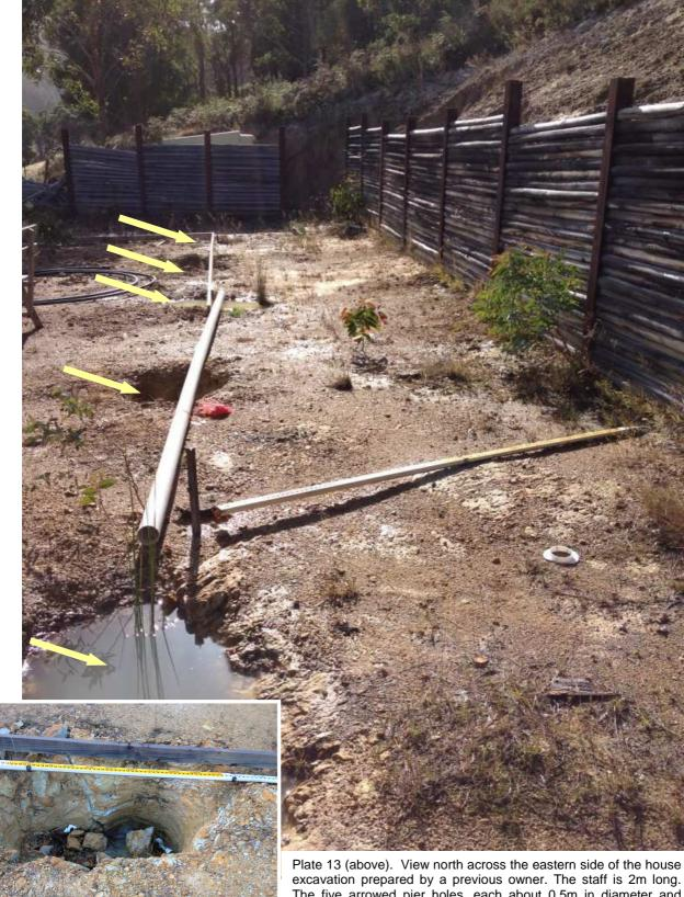
Plate 13 (above). View north across the eastern side of the house excavation prepared by a previous owner. The staff is 2m long. The five arrowed pier holes, each about 0.5m in diameter and ranging from 0.3 to 0.5m deep, were excavated in highly weathered Permian sandstone bedrock (inset at left). Bedrock is exposed over most of the foreground in this photo.
