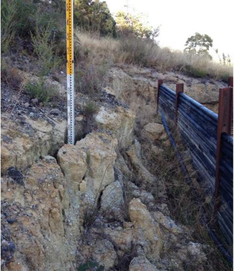
Plate 11 (above). View south at very small-scale rotational landsliding in colluvial soils at the southern end of the timber retaining wall.
