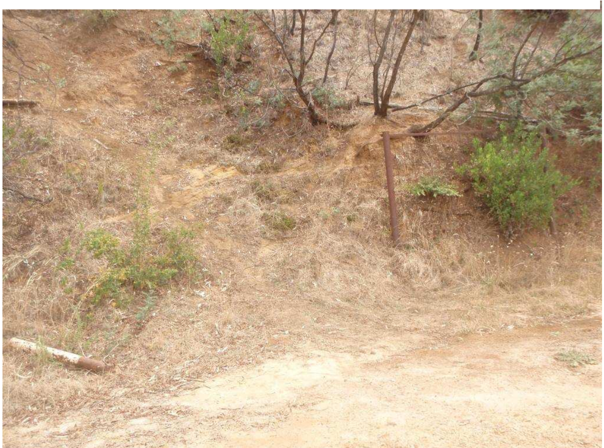
Plate 12 (below). Weakly cemented Tertiary sandstone exposed on the embankment where test pit L was dug.
