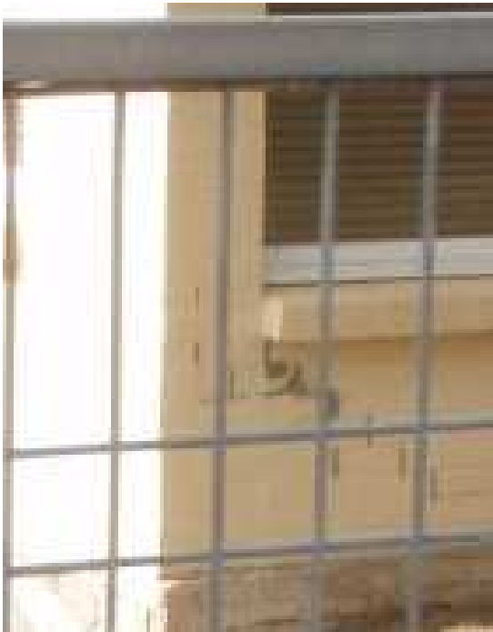
Plate 17 (below). Damage to houses in Thelma Street and Penquite Road probably caused by footing movement on reactive clay soils.
