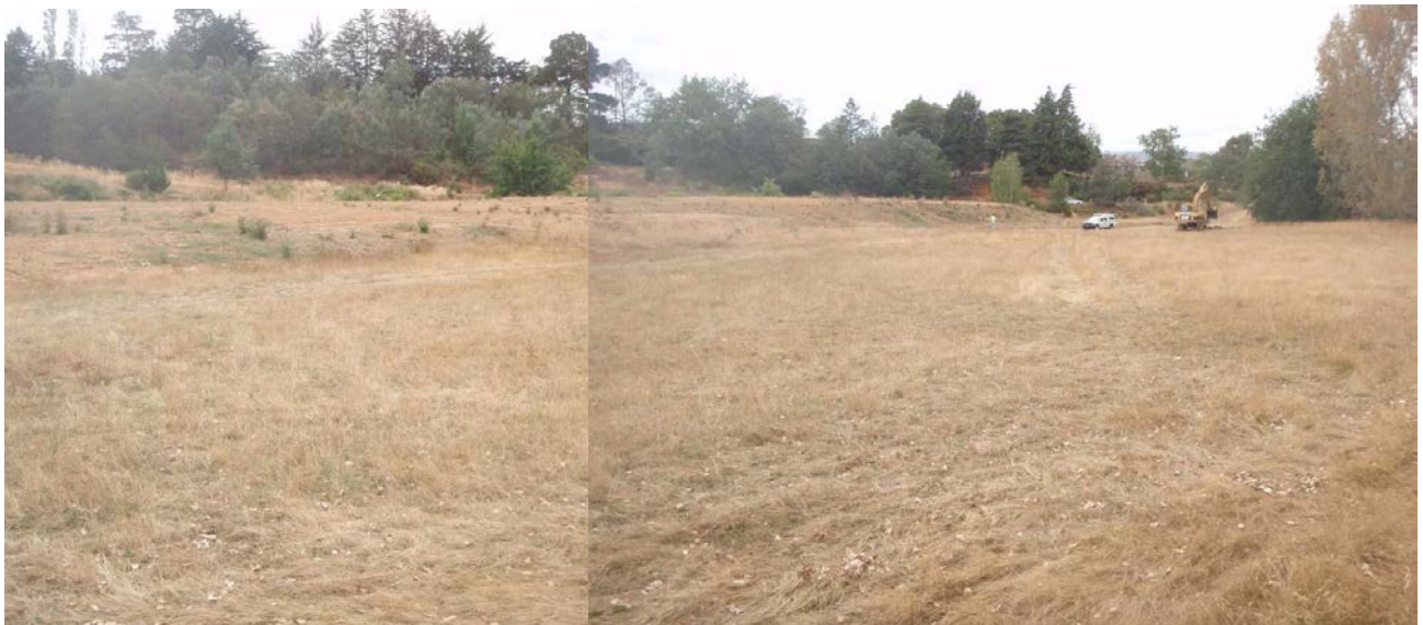
Plate 2 (below). A view similar to Plate 1, looking north. The excavator is digging test pit J. Most of the foreground will be raised a metre or more, and a metre or more taken off the mound, to create building allotments.
