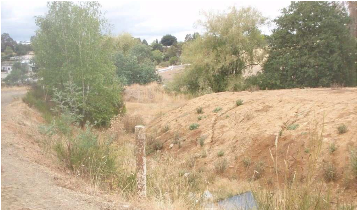
Plate 3 (above). View looking east showing raised fill at right on the former Eastman Oval, and the embankment at left.
