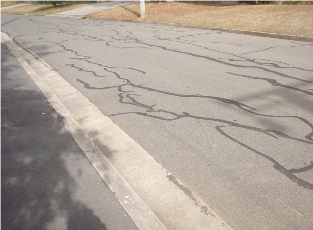
Plate 16 (above). Repaired cracking of bitumen in Thelma Street, which may have been caused by soil movement.
