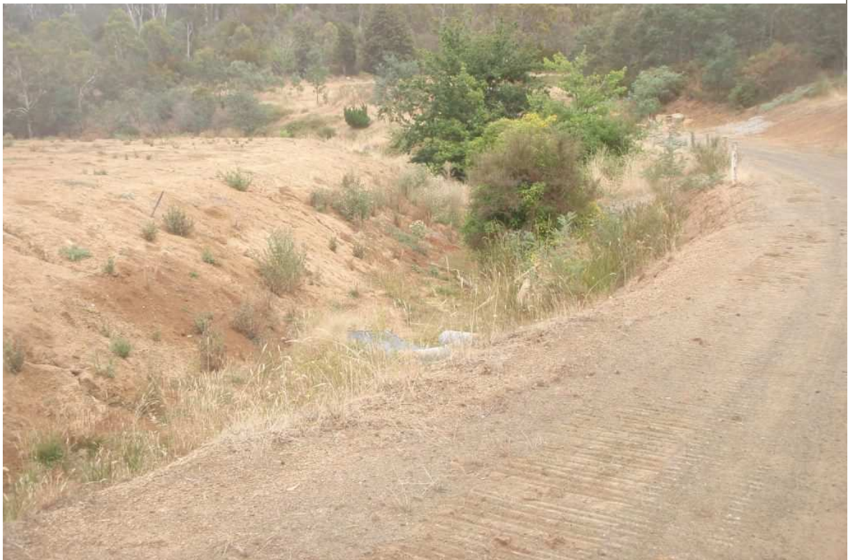
Plate 4 (below). Looking west from the same point as Plate 3. The raised fill is up to about 3 – 3.5m thick. The depression between it and the embankment will be filled in, and some of the mound removed, to create building allotments.
